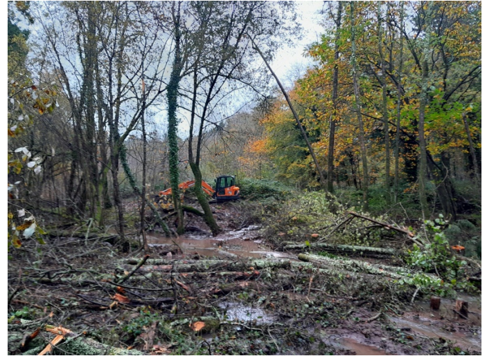
Installation of Natural Flood Management leaky dams in Cheriton Bottom, credit – Alex Shilling
